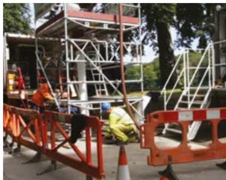
Once in-situ the liner is cured to the latest WIS specification using a steam or hot water boiler in combination with a liner coated with polyurethane or polypropylene for heat resistance creating a durable and successfully rehabilitated pipe with a life expectancy of over 50 years.
