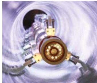
The UV sensitive resin impregnated liner is pulled into position using a winch, the light train is lowered into the liner and the end packers are fitted.
