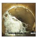
Cleaning of existing pipe by JetVac / Recycling unit.
